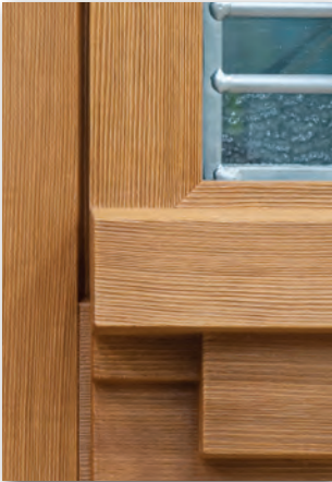
Details of the Craftsman Fir Grain Construction
